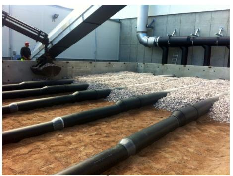
Figure – Bio Filter for  $30.000 \text{ m}^3/h$  off gases for a waste incineration plant in Västervik, Sweden during construction.
