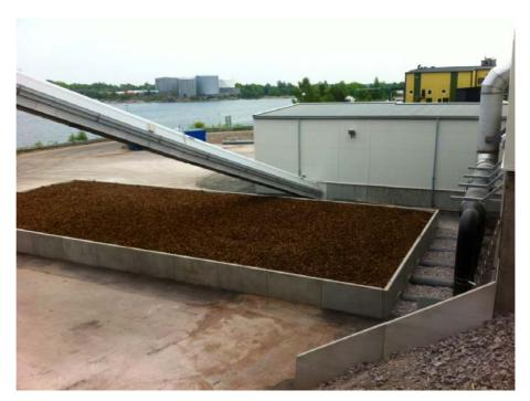
Figure – Overview of the Västervik filter. This plant is situated by the sea some 250 meters from a residential area in the idyllic town of Västervik. Before installation of this filter, there where massive complaints of odour from an elderly installation.
