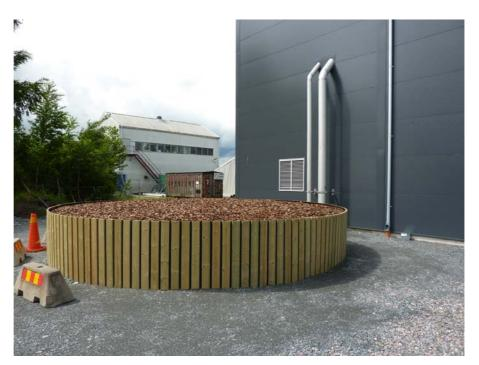
Figure – Small bio filter for cleaning of carcinogenic trimethylamine from a plant for modified starch for the pulp and paper industry in Sweden. This filter is stage to accept various operation modes. It will accept flows from  $400 - 2000 \text{ m}^3/h$ .
