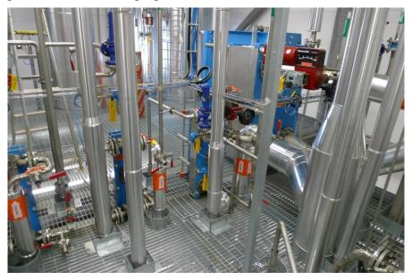
*Photo – Part of raw distillery process plant. The whole distillery building is classified according to Atex regulations.*
