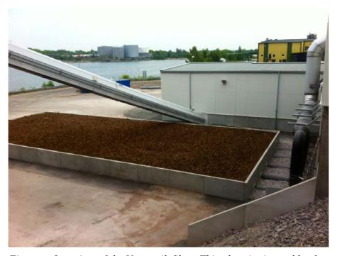
Figure – Overview of the Västervik filter. This plant is situated by the sea some 250 meters from a residential area in the idyllic town of Västervik. Before installation of this filter, there where massive complaints of odour from an elderly installation.
