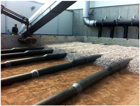
Figure – Bio Filter for 30.000 m³/h off gases for a waste incineration plant in Västervik, Sweden during construction.
