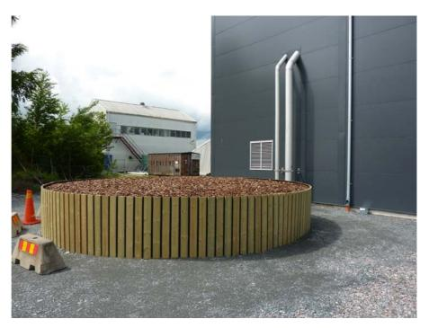
Figure – Small bio filter for cleaning of carcinogenic trimethylamine from a plant for modified starch for the pulp and paper industry in Sweden. This filter is stage to accept various operation modes. It will accept flows from  $400 - 2000 \, \text{m}^3/\text{h}$ .
