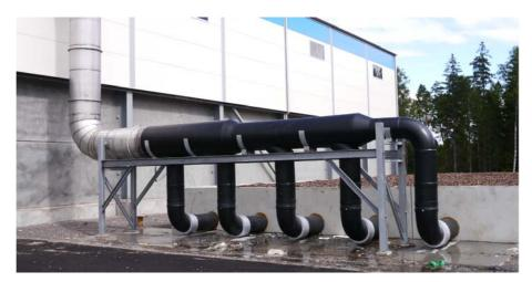
Figure – Polluted air from fuel storage/preparation at the waste fired plant in Nybro. The capacity is  $30.000 \text{ m}^3/h$ .
