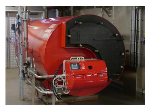
*Photo – Gas burner mounted on the hot water boiler*
