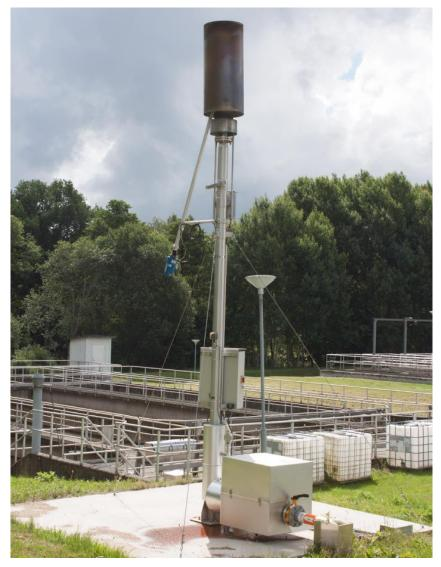
Photo – Rebuilt open flare
