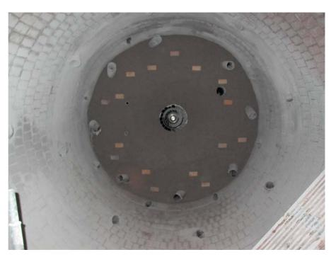
$Figure-refractory\ lining\ of\ adiabatic\ incinerator.$
