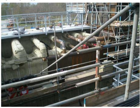
Figure – Erection of 30 MW<sub>th</sub> boiler for saturated steam. In this case it is an outdoor installation (Stenungsund)
