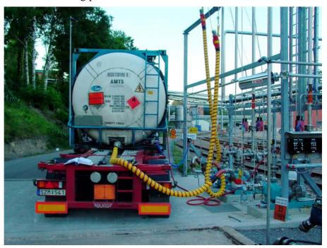
Figure – Receiving station for hazardous waste.
