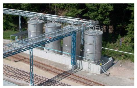
Figure – Storage tanks for hazardous waste. Several different types can be mixed simultaneously.
