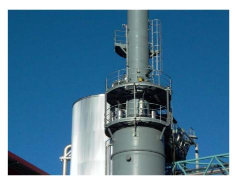
Figure – Exterior of combine scrubber and wet electrostatic precipitator. This unit is built in GRP/epoxy and is 65 meters high but can be built lower (Perstorp)
